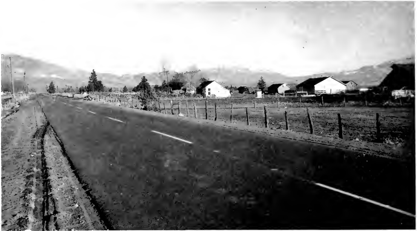
View of recently completed FAS Route 1166, in Siskiyou County, showing typical farm area served
